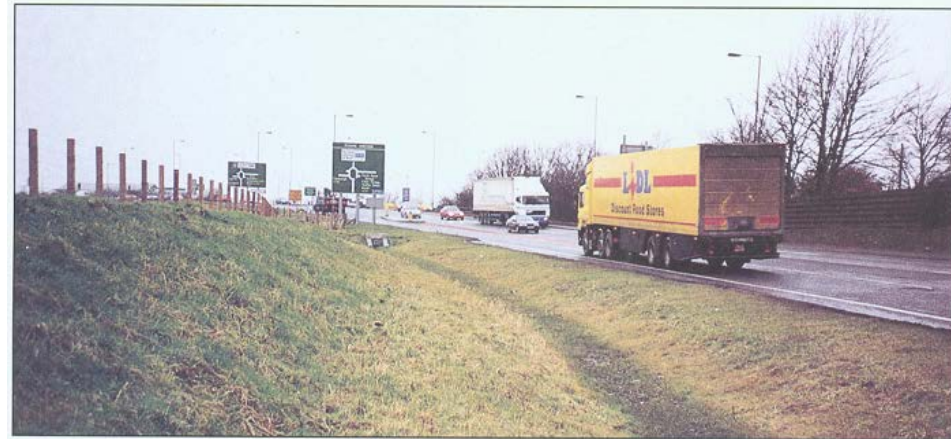
Swale on A8000 near Edinburgh. No kerbs or gullies are required.
